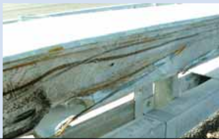
Adjoining concrete step barrier and steel barrier post-lorry impact on M6. The steel barrier sustained significant damage, needing replacement.
