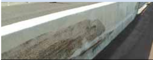
Adjoining concrete step barrier and steel barrier post-lorry impact on M6. The steel barrier sustained significant damage, needing replacement.
